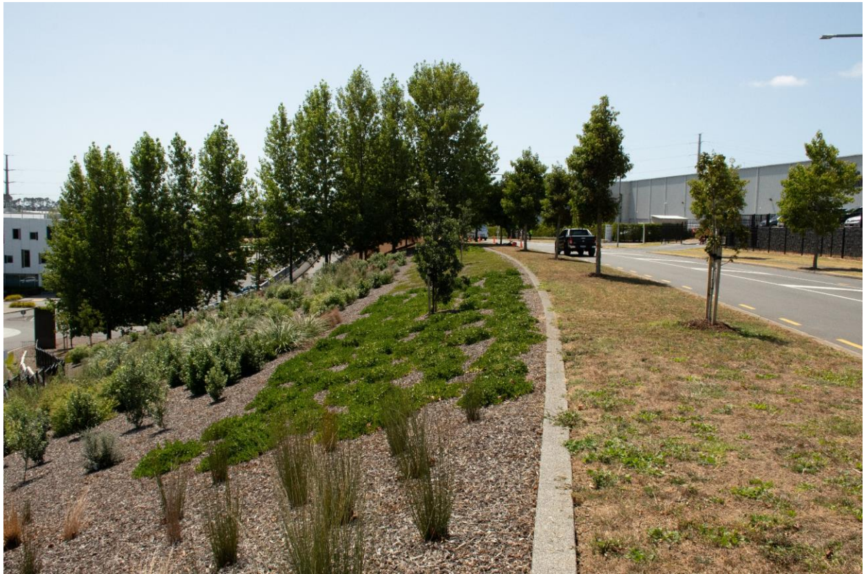
Image 3: Highbrook Business Park - Batter Slopes to accommodate gradients and create building platforms
