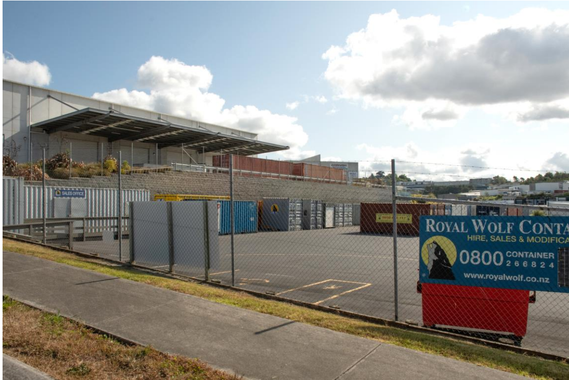
Image 5: Ingot Place, Silverdale – Use of retaining wall to manage approximate 4m height differential between sites.
