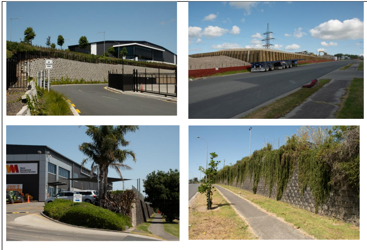
Image 6: Clockwise from top left: crib wall, timber pole, keystone wall, concrete with rock face
