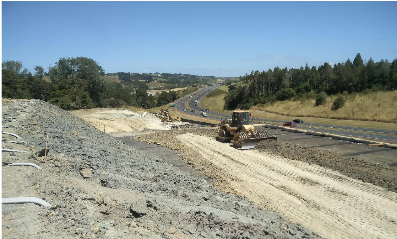
Image 2: Highgate Business Park, Millwater – considerable earthworks were undertaken to manage pre development slopes in excess of 20%
