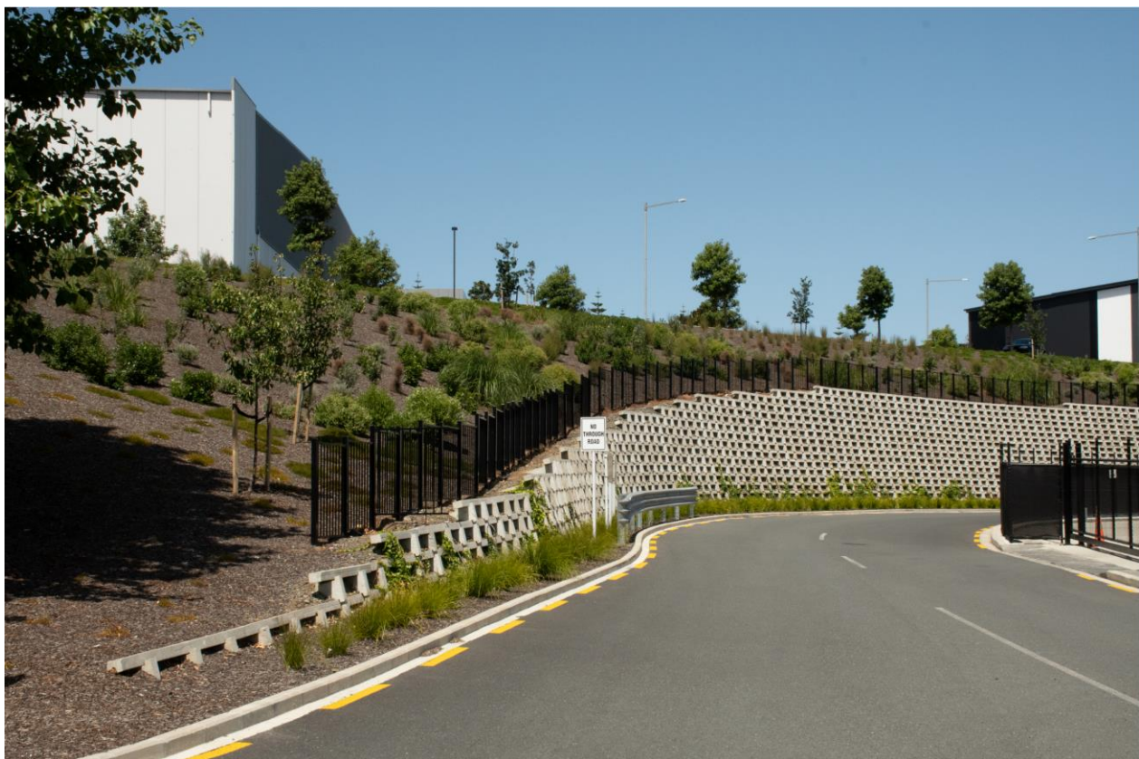
Image 4: Highbrook Business Park – use of batter slopes and retaining walls to accommodate a 10m height differential.
