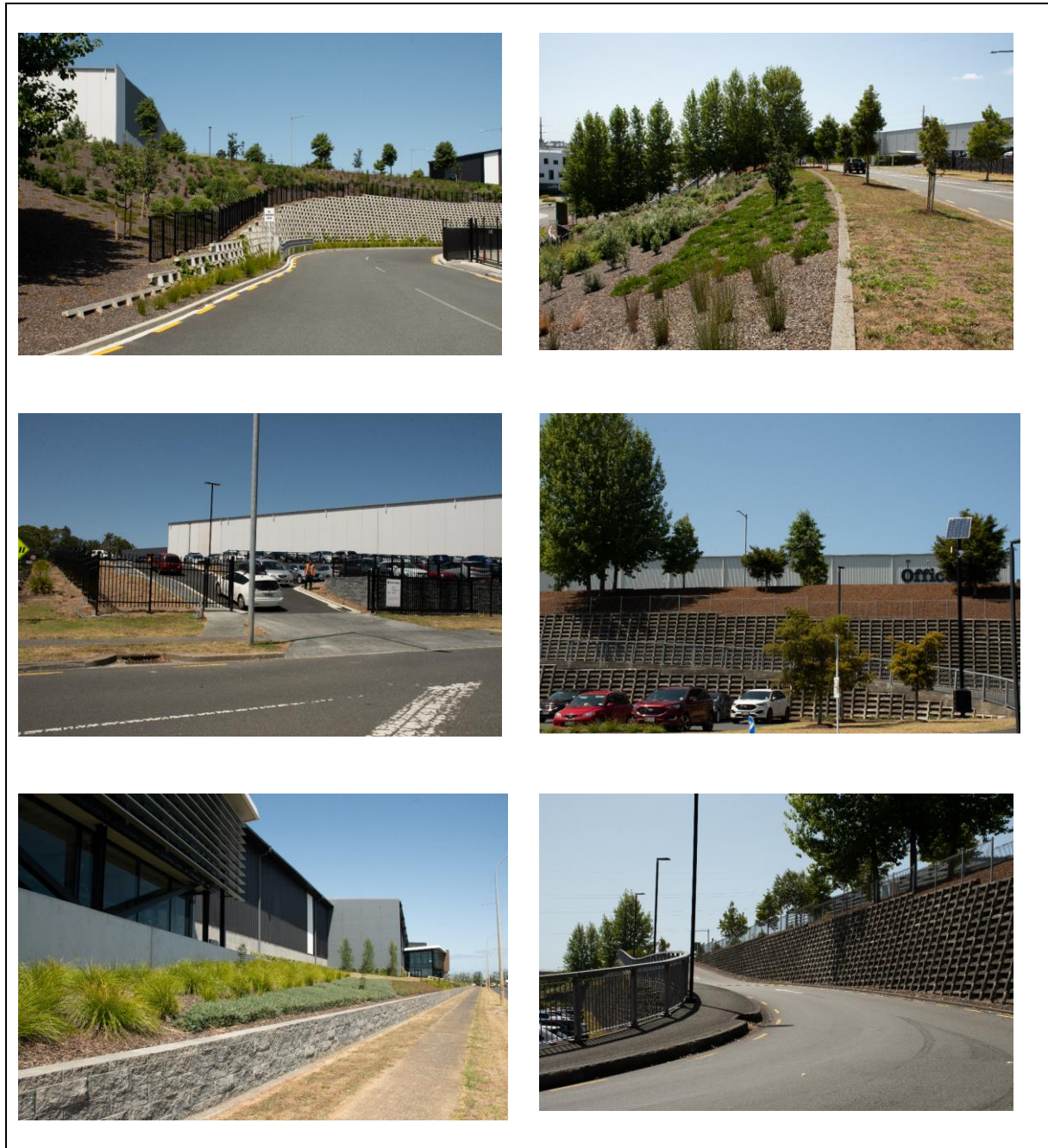
Image 7: – Combinations of retaining walls, roading and batter to manage changes in levels
